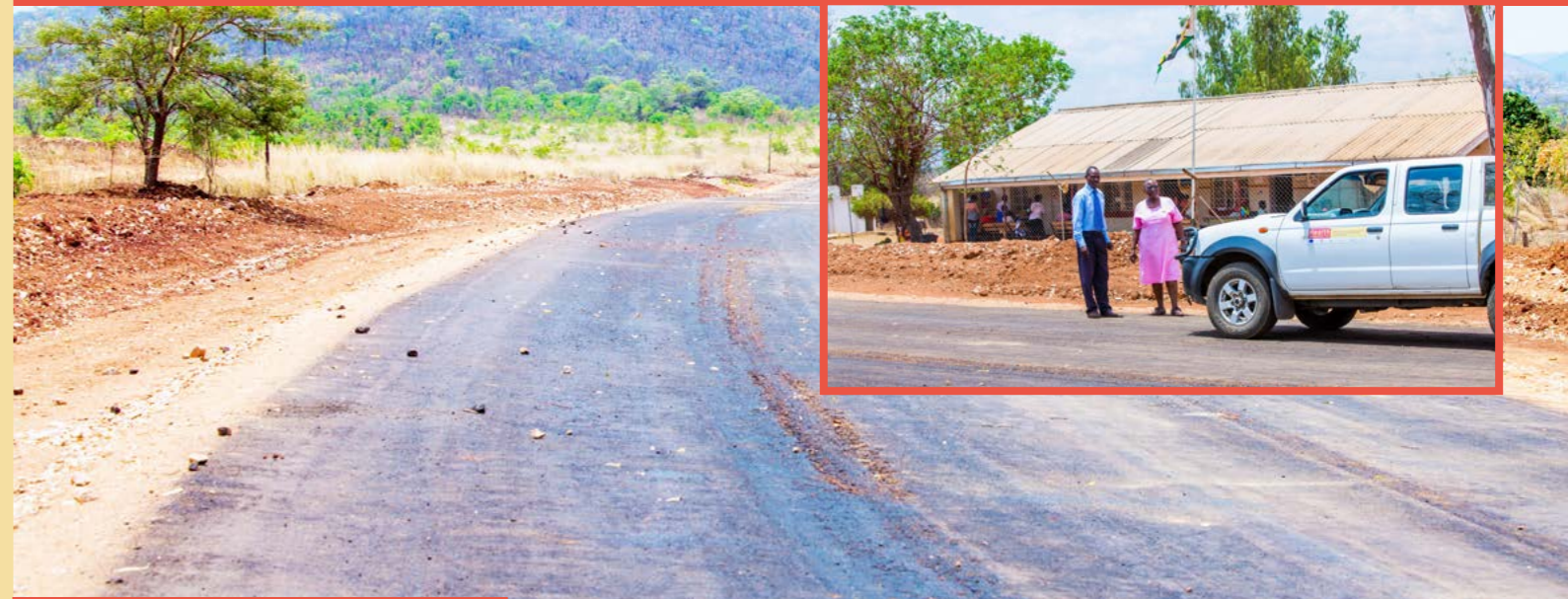
Matepatapa road under construction
